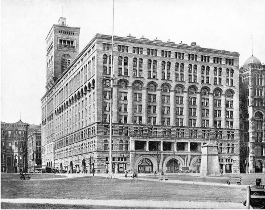
Figure 1 Chicago's Auditorium Building, c. 1889. The tower marks the entrance to the theater, while the three arches facing the park offer entry to the hotel. Photo from America from Alaska to the Gulf of Mexico, Series 1 , ed. G. R. Cromwell (New York: James Clarke, 1894).
